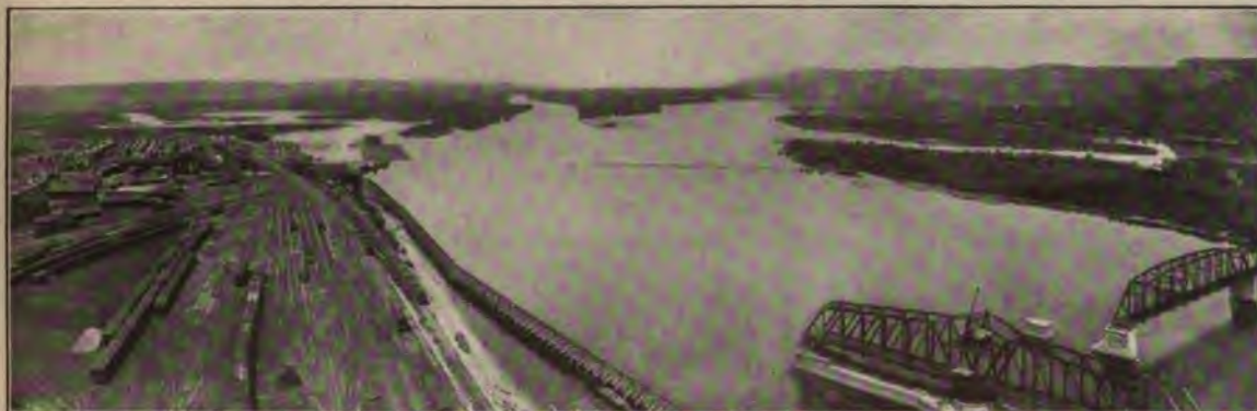
The Mississippi River and its flood-plain at Winona, Minn., looking up the river. Notice the drawbridge which is drawn to permit steamboats to pass and the jetty on the left-hand side to deepen the channel and prevent the banks from being washed away. Above notice the several branches, all of which are a part of the river. The opposite shore is Wisconsin.
